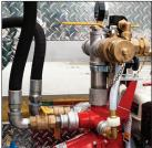
Pump features stainless steel piping & brass valves
